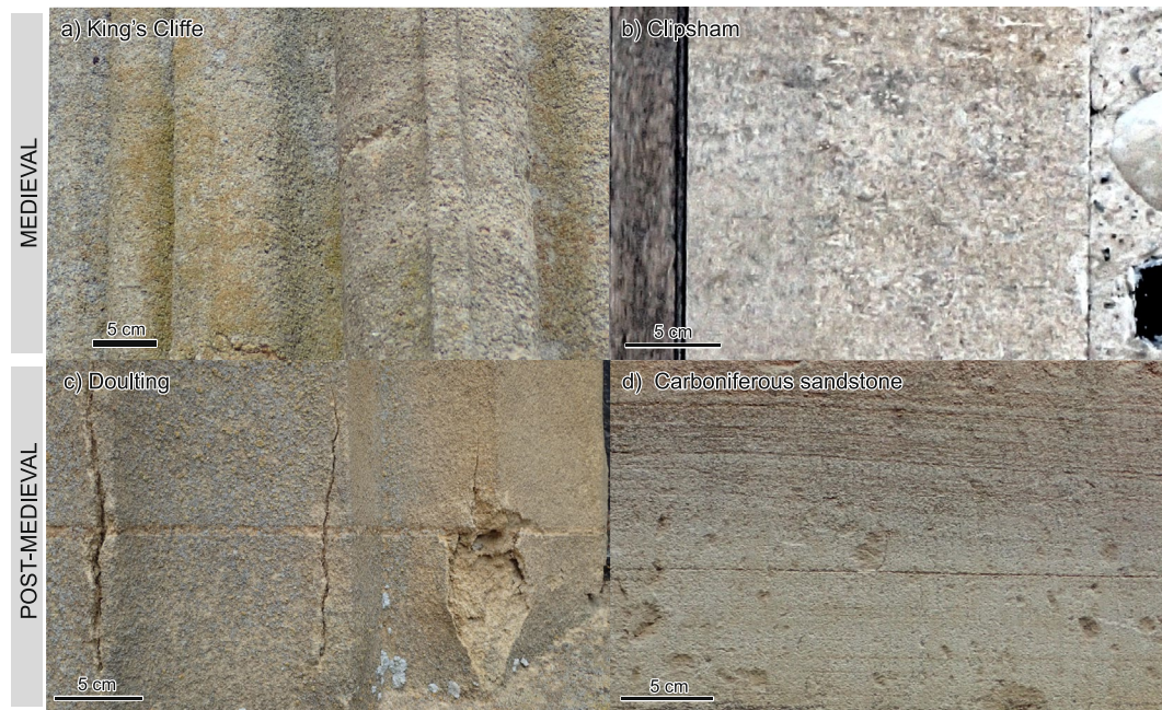
Fig. 6 Imported stones ( italicised ) infrequently used in the study area: a) ? King's Cliffe , Fenstanton St Peter & St Paul, 1345–52 chancel east window; b) Clipsham , Great Abington St Mary, north porch,
