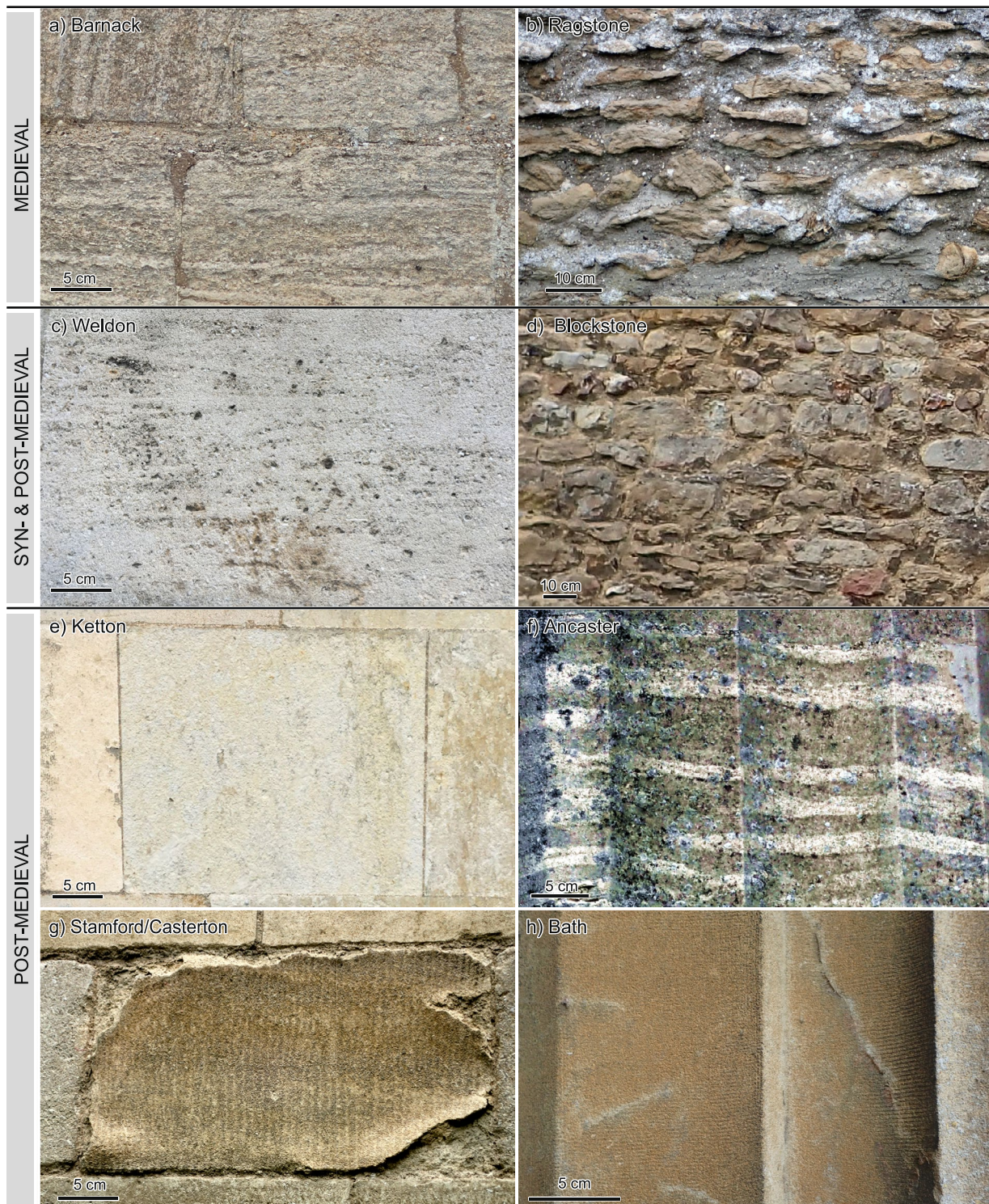
Fig. 5 Imported stones ( italicised ) commonly used in the study area: a) Barnack ashlar, Stourbridge St Mary Magdalene, later C12 chancel south; b) Ragstone rubble, Swaffham Prior St Mary, C15 north aisle; c) Weldon ashlar, Cambridge St Mary the Great, 1491–1550 tower west; d) Blockstone (oolite and Clunch) rubble, Willingham St
