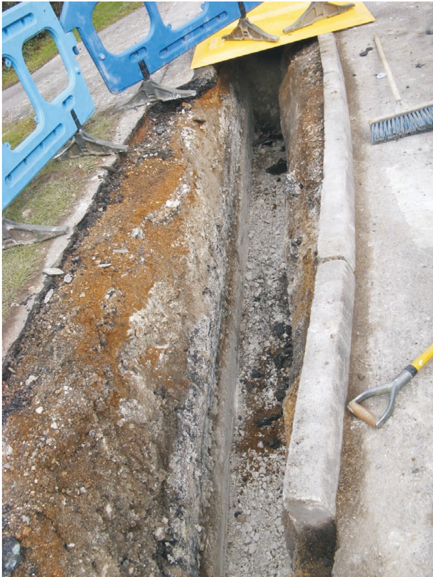
Figure 3. Pipeline cross-section
