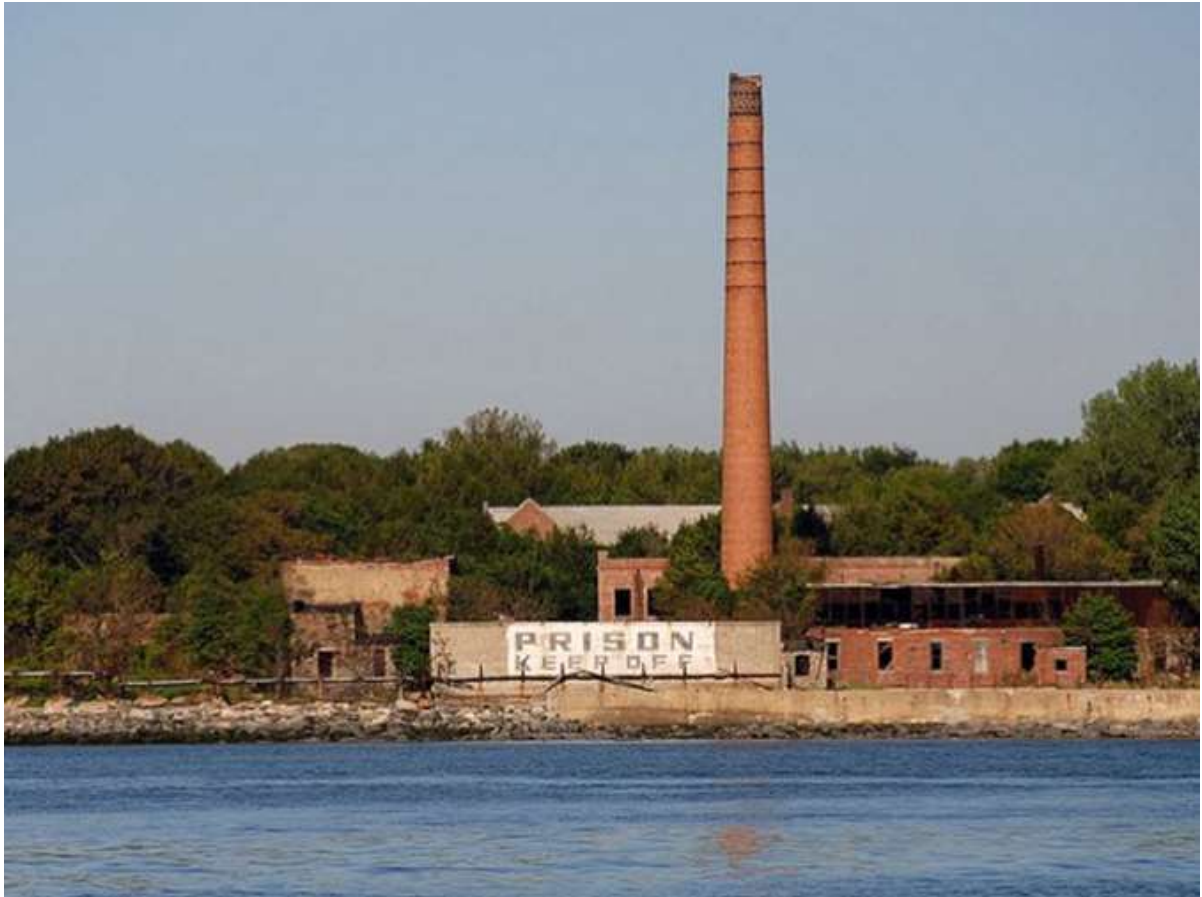
Figure 8. Eastern seawall of Hart Island 28 October 2010. (Credit: Janko Puls, Flickr).
