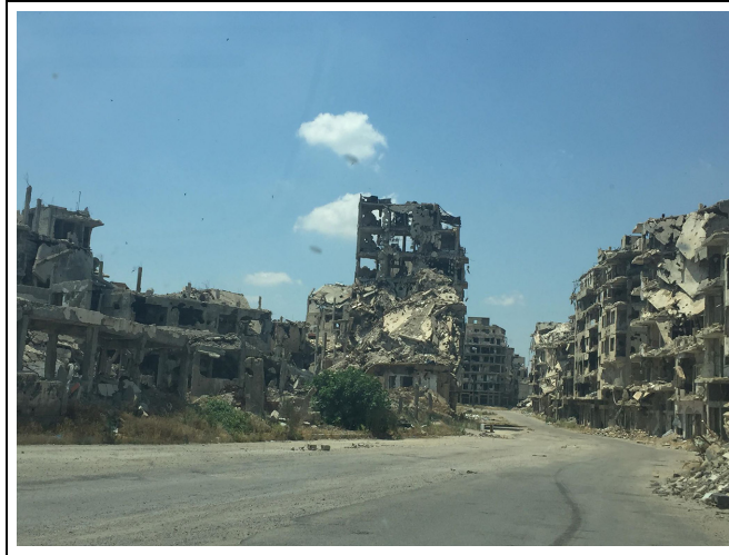
Figure 1. Destruction of Homs.
