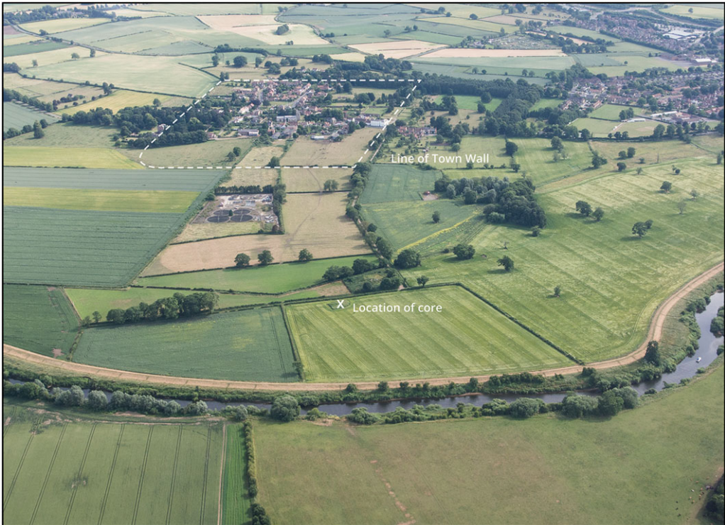
Figure 2. Aerial photograph of Aldborough showing the extent of the walled town and the location of the sediment core (figure by D. Powlesland & V. Herring).
