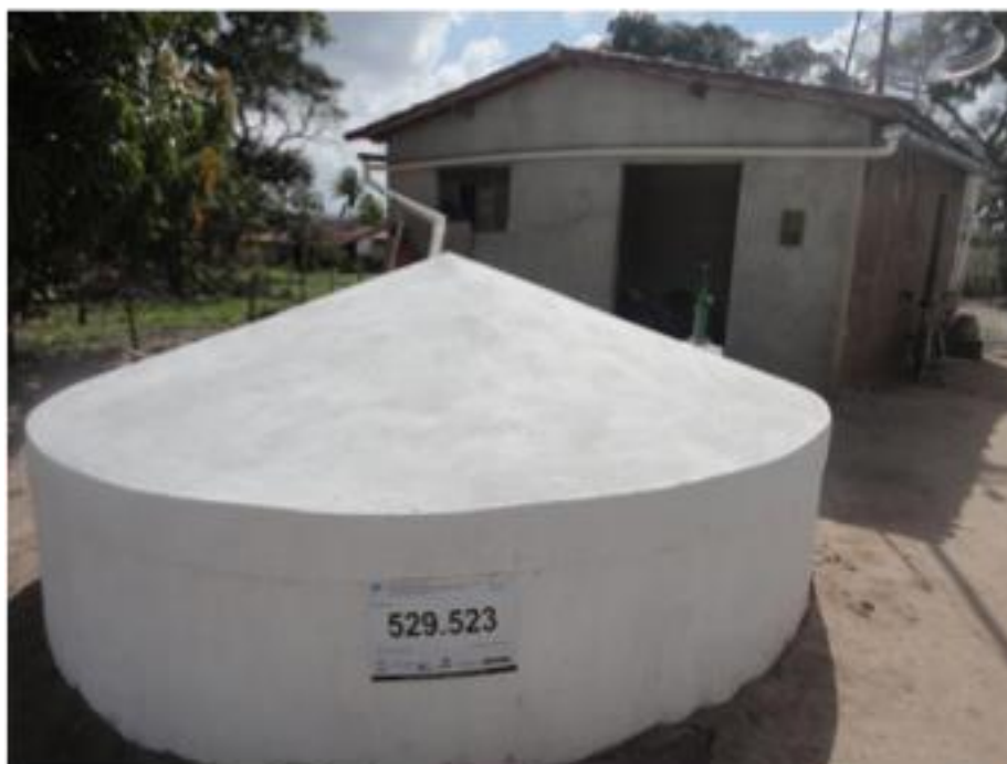
Figure 3: Concrete Cistern of 16,000 liters
