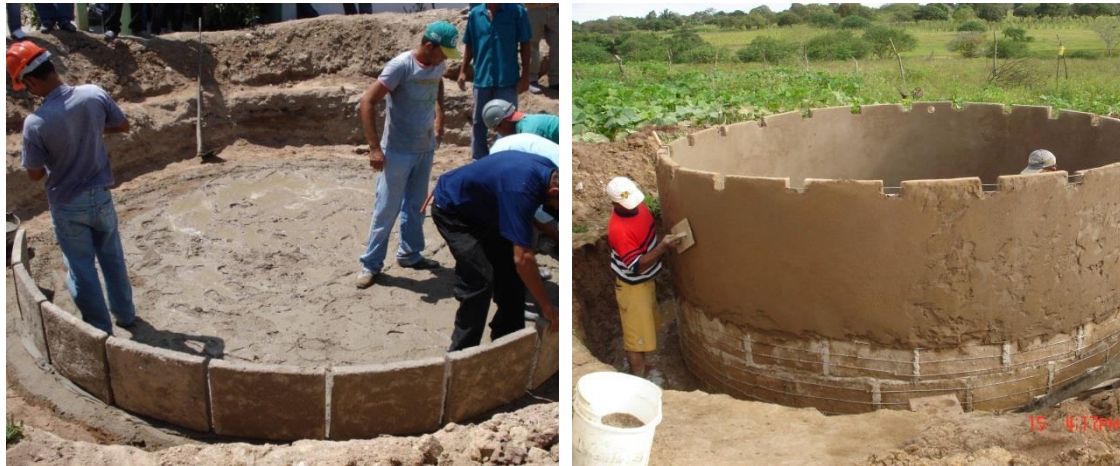
Figure 4. Community building a concrete cistern
