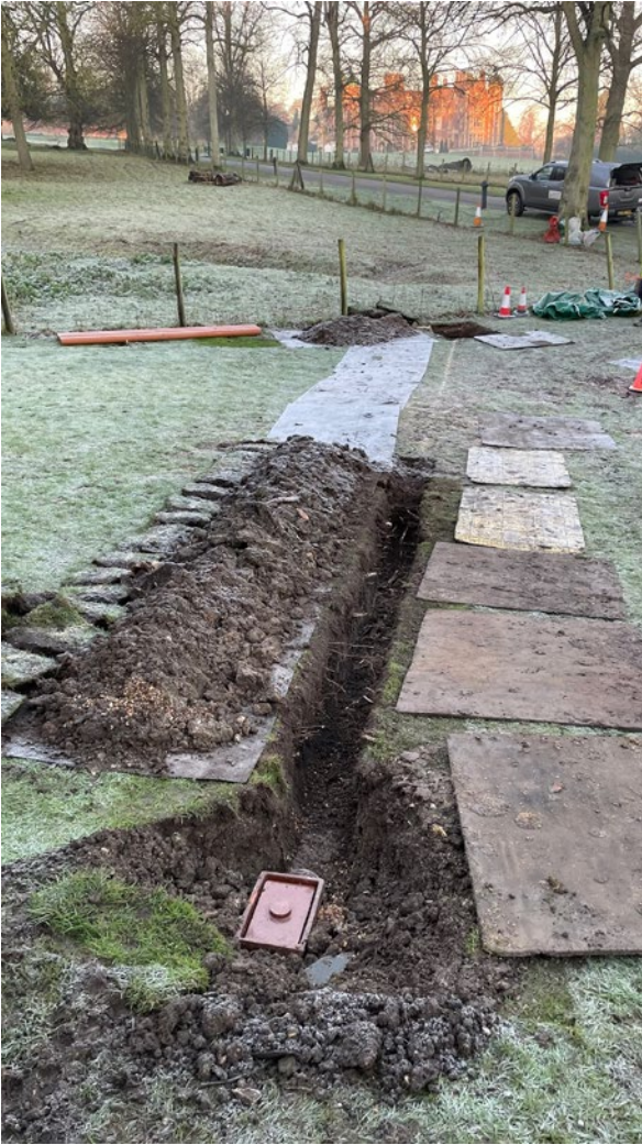
Figure 3. Northern segment of the trench, looking NW
