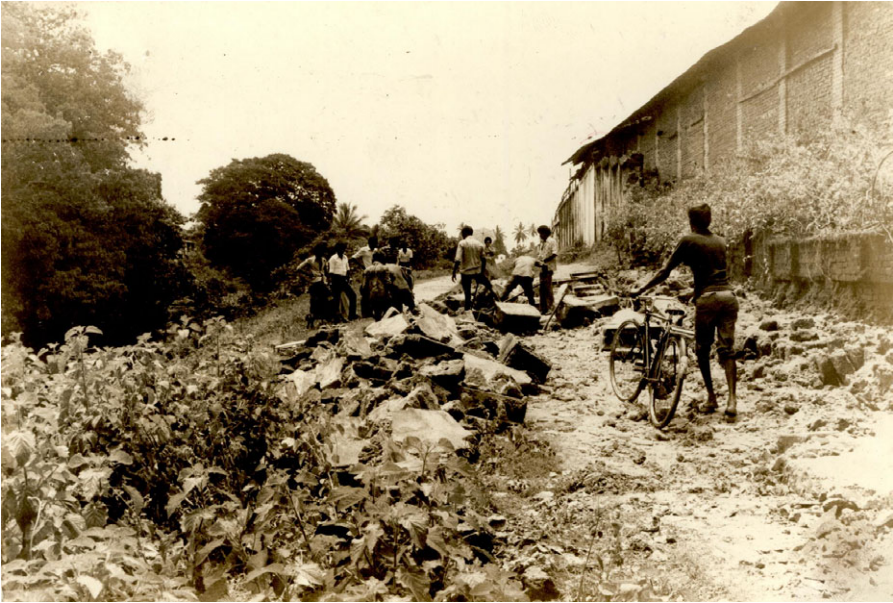
Figure 5. 'The twenty foot wall of the Wellawatte Spinning and Weaving Mills which collapsed' (24 May 1984), Times Collection. Reference Code: 326-IM-0061-0171. With permission from the Sri Lanka National Archives.
