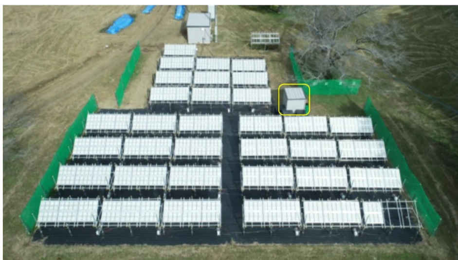
FIGURE 10 | An overhead view of the 100 m 2 solar hydrogen production system. Reproduced with permission [64], Copyright 2021, Springer Nature.
