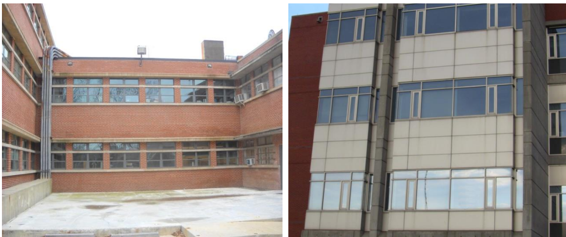
Figure 3: Two building façades for multi-step stereo camera calibration experiments
