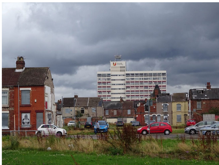
Figure 1: A photograph taken during fieldwork in 2019, showing partially demolished streets in Gresham in front of a nearby Teesside University building, several years after the plans for demolition in Gresham under HMRP were announced
