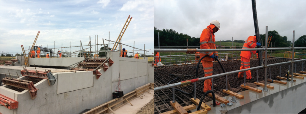
Figure 6. Bridge under construction during deck casting
