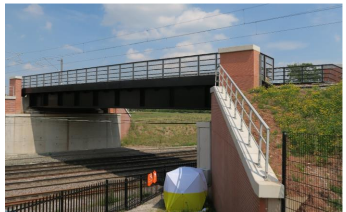
(a) Intersection Bridge 5
