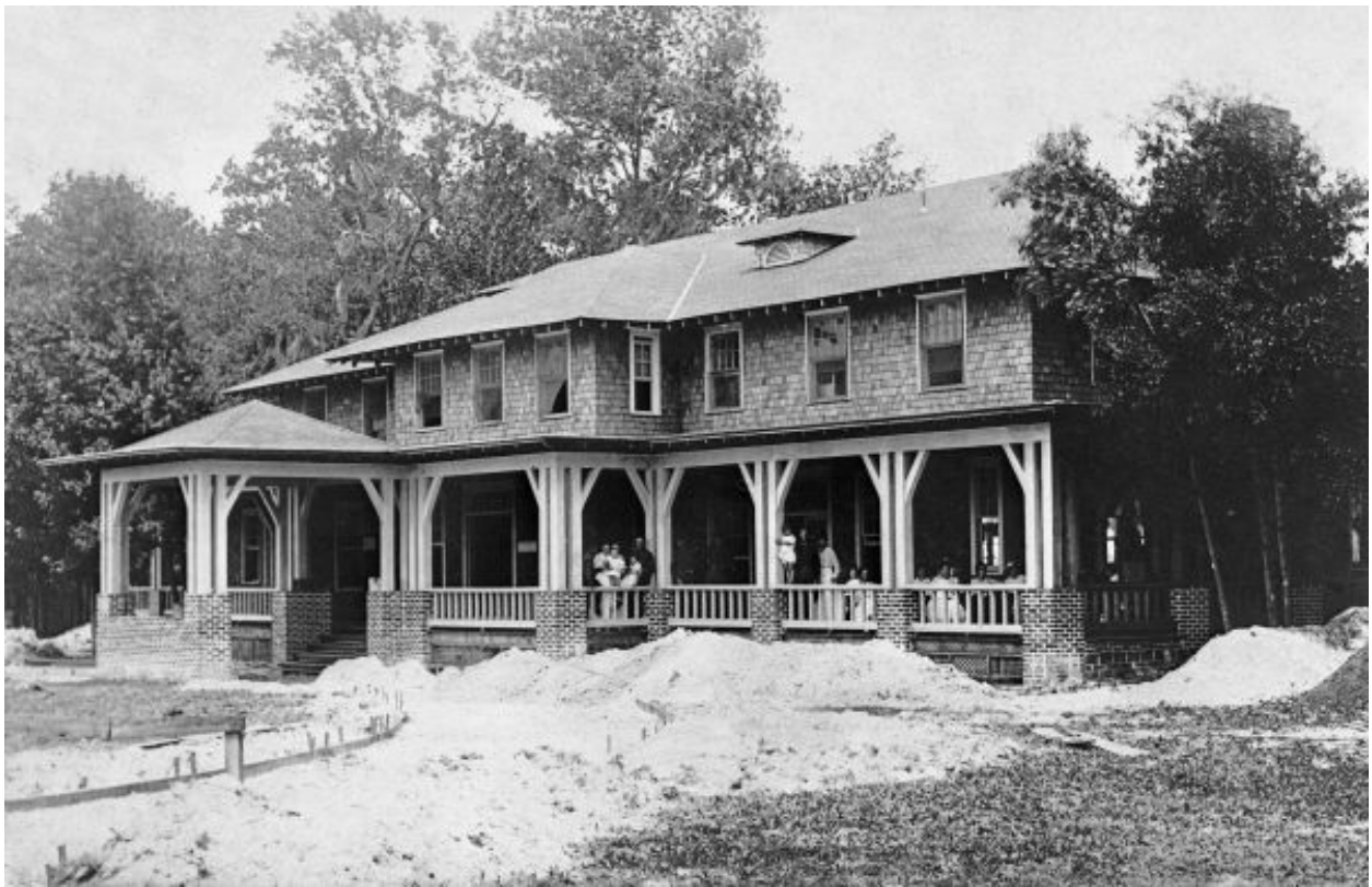
Figures 2.15 & 2.16: These ca. 1918 images of the YWCA Hostess House at Camp Johnston in Florida show the lengths that the YWCA went to bringing domestic-style architecture into the training camps. For more extensive imagery of the Hostess Houses, see Brandimarte, “Women on the Home Front: Hostess Houses During World War I.”
