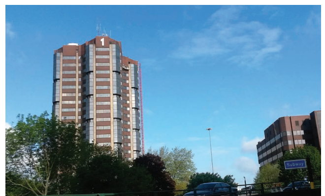
Figure 5. One Hagley Road during internal construction work
