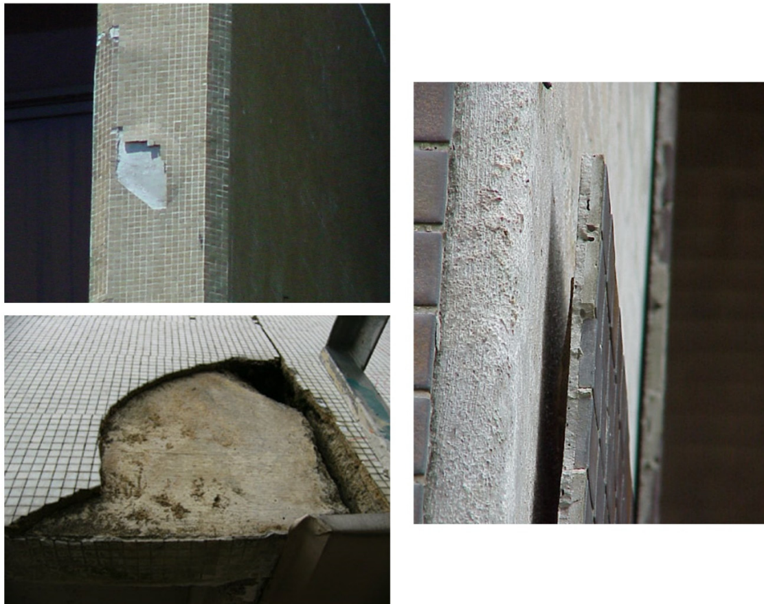
Figure 10. Debonding of mosaic in a patch.
