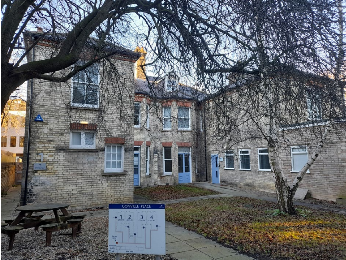
Figure 26. Back of 1–2 Gonville Place. Looking NW
