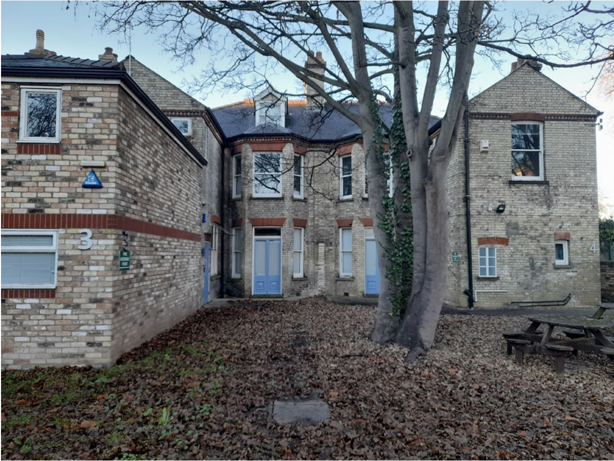
Figure 27. Back of 3–4 Gonville Place. Looking NW
