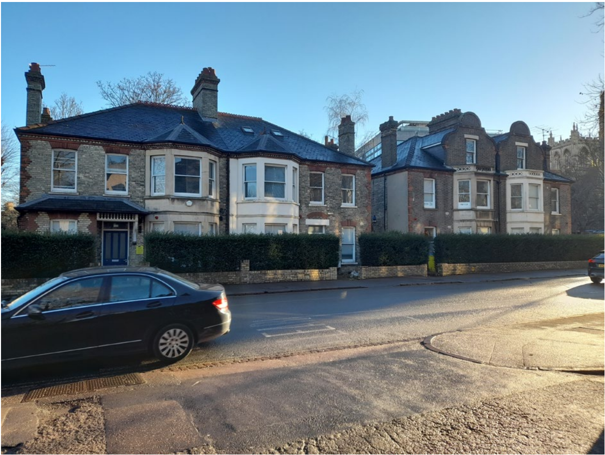
Figure 19. 1–4 Gonville Place, looking S
