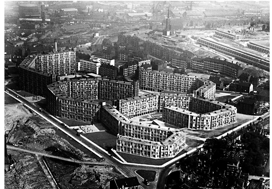
Fig. 1. Park Hill, Sheffield, Jack Lynn and Ivor Smith, completed in 1961, photograph of 1969 by Bill Toomey (RIBA Collections)
