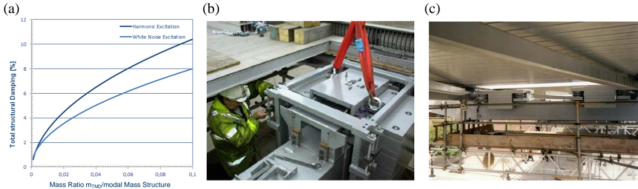
Figure 2: (a) typical additional damping vs. mass ratio achieved for random and harmonic excitation; and installation of (b) laterally- and (c) vertically-acting tuned-mass absorbers on the Millennium Footbridge.
