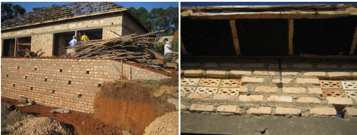
Figure 5: Mortar thicknesses of up to 30mm is normal for brick walling (Uganda)
