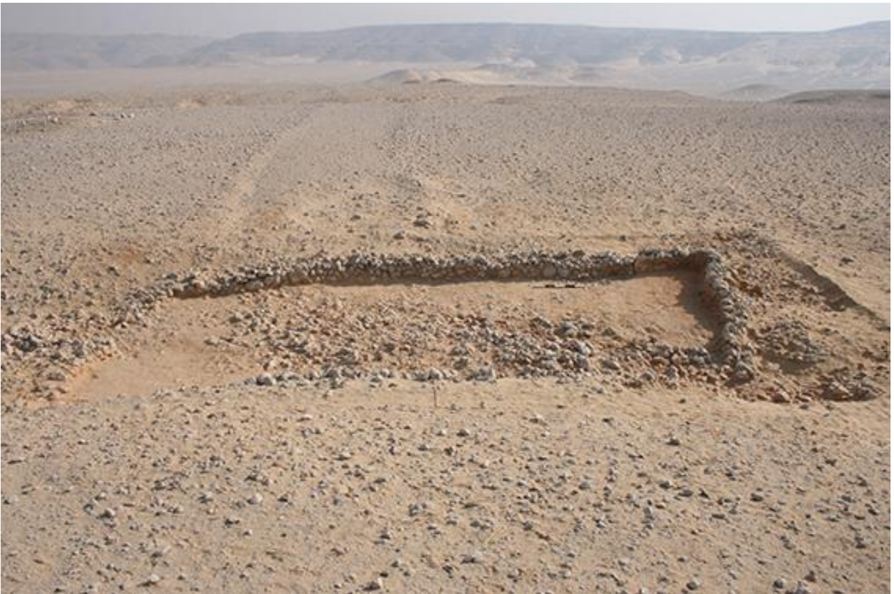
Figure 3. Structure I after excavation, facing north-east. Image courtesy of the Amarna Project.
