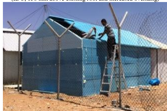
h) XPS insulation and roof shade
