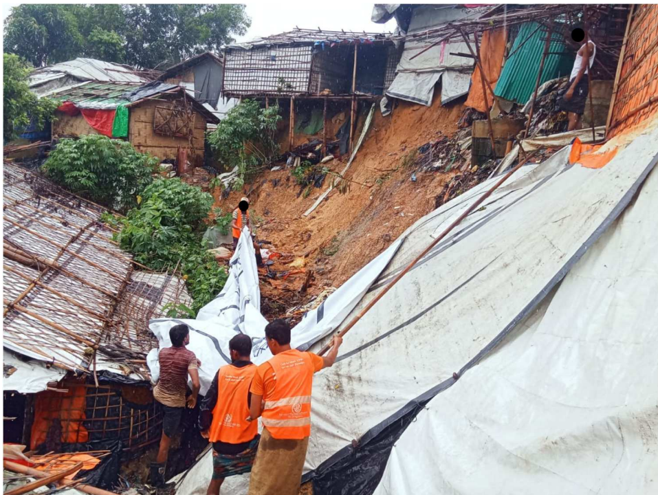
Figure 2. Shelters are built on top of uneven and risky slopes.
